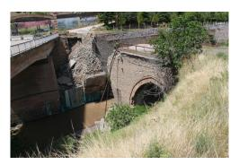
Figure 7. Elazığ-Maden Bridge, part of which was destroyed due to flood and overflow (Authors archive, 2023)
