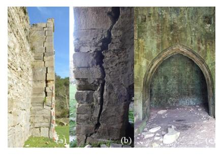
Figure 10. Problems in building scale; crack and splitting in main portal (a) and portico pier (b) discoloration and microflora in shelter (c)
