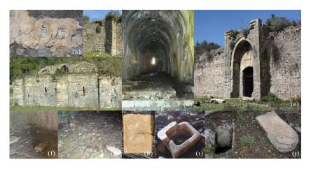
Figure 8. Values in building scale; plaster mason signature (a), triangular butress (b), relieving vault in shelter roof (c) platform design (d), south facade with different stone usage and portal design (e), latrine design (f), room with tandır remain (g), authentic roof tile (h), yemlik remain (ı), illumination hole with closing stone (j)
